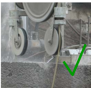
Position slack side pulley outside of concrete.
