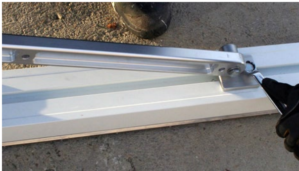
d. Tighten the upper bolt loosely.
